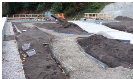
Paths and planting areas during the landscaping works.
