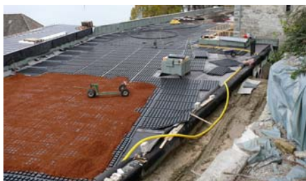
The drainage and water storage element Floradrain® FD 60 makes sure that the overall roof area is being drained properly via its two narrow edges.
